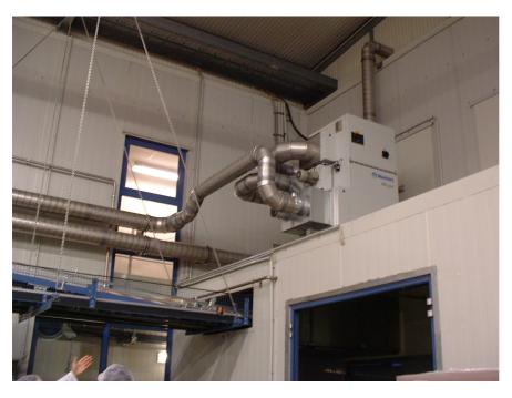
Within the spiral freezer, the product itself brings humidity, and due to the wide difference in temperature and pressure between the ambient air and that in the freezer, warm, moist air streams into the -40°C freezer through the openings, through which the product is fed. The result is frosting and icing up of the conveyor belts and refrigeration components, causing frequent interruptions to defrost and clean the plant.
