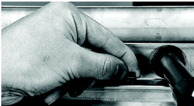
Figure 4.4 Open the safety catch on the distribution header by turning a quarter turn
