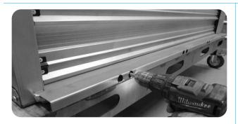
Fix the lower hook to the bottom panel by means of 4 self-tapping screws (round head - 6.3x19).
