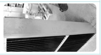
Place the additional frame on the side panel and fix it by means of 3 self-tapping screws (4.2x19).
