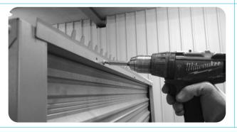
Remove the safety mesh and then install the upper hook on the top panel by means of 4 self-tapping screws (round head - 6.3x19).
