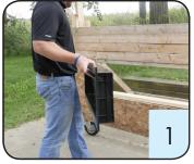
Place the inlet into framed opening. NOTES: the opening size is critical! Leave always a gap of 0.2inch or 5mm evenly distributed around the unit.
