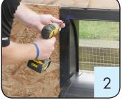
Fasten the left and right lateral side support using appropriate screws (2-inch or 5 cm). NOTES: Fastening points are marked on both supports. Screws and fittings are not included, Choose screws and fittings that are suited to the material in the wall and have sufficient holding power.
