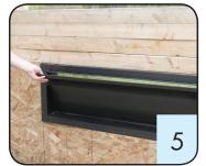
Verify the correct movement, opening and closing of the inlet.
