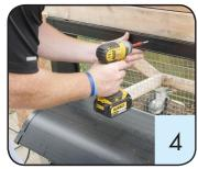
Push slightly up on the top header center, 0.25 inch or 0.6 cm. needed difference. Fasten the top header profile using appropriate screw. NOTES: Make sure the slight curvature of approximately 0.25 inch or 0.6 cm is achieved before fastening. Fastening should be done in the center, on the marked line.
