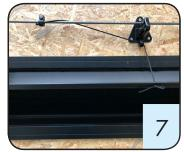
Install a small pulley at the top of the inlet. NOTES: Pulley or fitting are not included.
