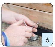
Fasten the (2) L-Screw hooks evenly spaced above header. Place 0.5 inch or 1.2 cm above the top header, opposite to the direction of pull. NOTES: Avoid interference with the
