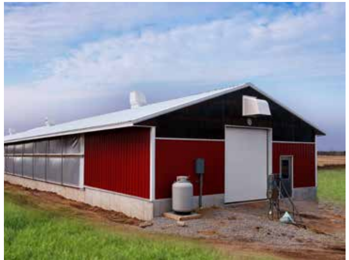
Ridge Fans & Fiberglass Weatherhood
