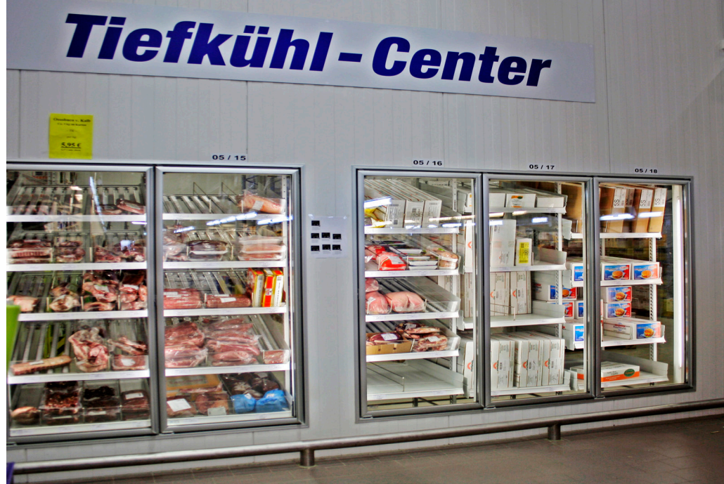
The employees working in the -15°C cold store enjoy safe working conditions with dry floors free of ice, no formations of fog or ice build-ups on doors, products and ceiling.
