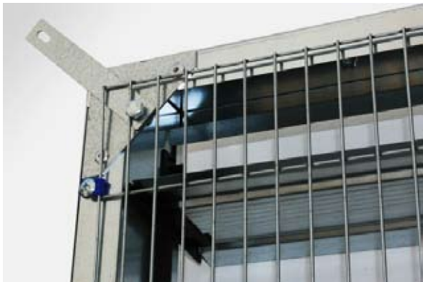
SMT fitted with guard mesh to prevent wild animals and birds from entering.
