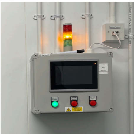
Traffic light system in the air lock protects conditions when entering and exiting.
