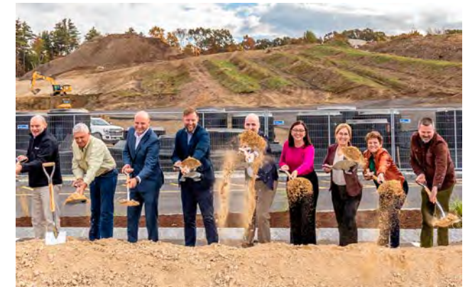
The first shovel was put in the ground in Amesbury, USA
