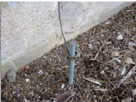
Figure 26: Ground Connection
