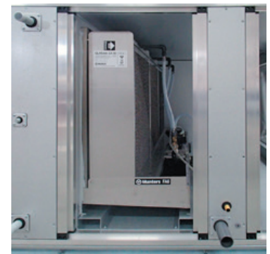
Example of an FA6 installation in a section of an air handling unit
