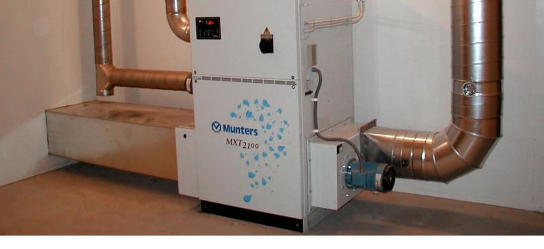
Films are stored in stable 5°C conditions, and 30% relative humidity. The films were previously stored in a warehouse, which had a cooling system meant to provide proper temperature and humidity. However, the relative humidity could not be kept sufficiently low and constant all year round.
