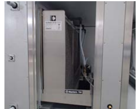
Example of an FA6 installation in a section of an airhandling unit
