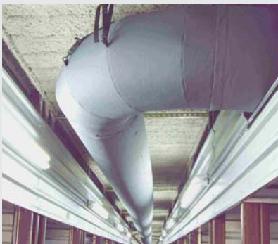
Dryflo is flexible, unlike metal ducting.
