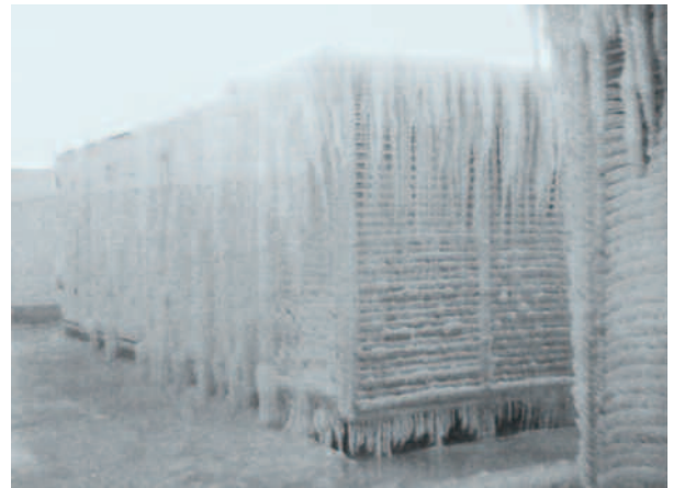
Conditions do not always have to be 'extreme' for extreme problems to arise. These images of totally ice-bound air intakes were taken in northern Germany in ambient conditions of around 0 °C.
