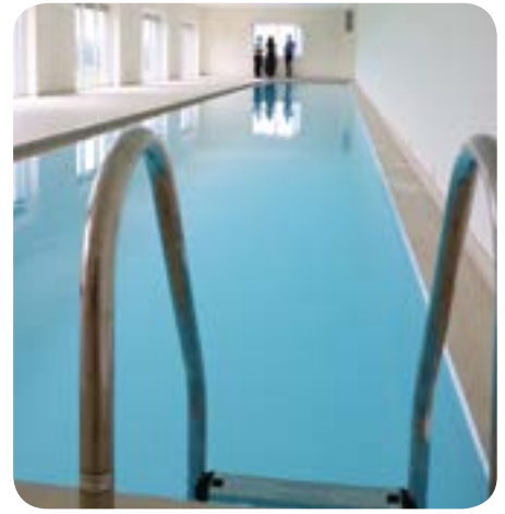
The Fitness area's pool is designed to act as a water supply back-up for the Oasis™ units in the unlikely event of a disruption of the public water supply.
