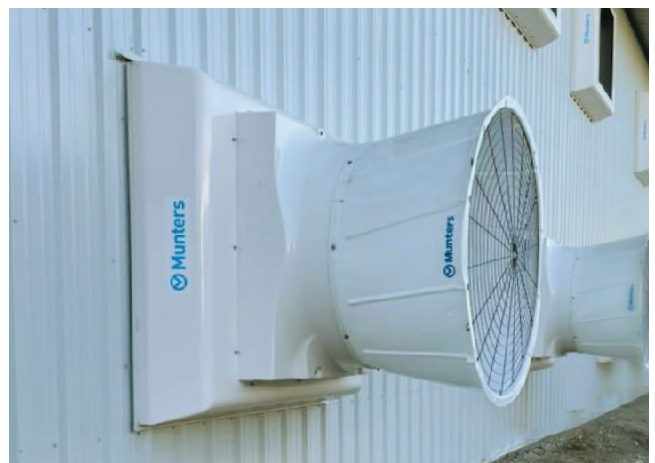
LTX Housing installation in Rising City, Nebraska
